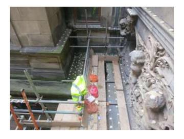
Scaffolding having been erected, all the ledges at the top level of the scaffolding (level 5) were treated with *Bird Free.* Roosting spots on the ornate stonework were also treated, as were the ledges above the stonework (above right). The wide ledge level with the scaffolding to the south was treated with three rows of dishes, as eggs had been observed there.
