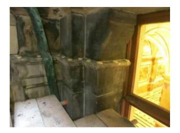
At level 3, the balustrade and floor of the balcony inside the recess to the north were treated with Bird Free. (The floors of the balconies were nesting sites, so the dishes were fixed at 250mm centre to centre.)
